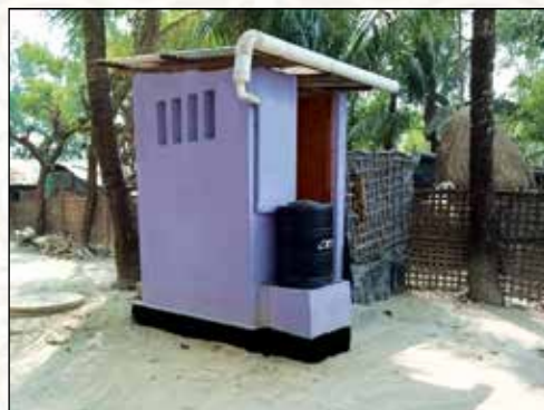
Latrine installed by DPHE at Ashrayan Community.
